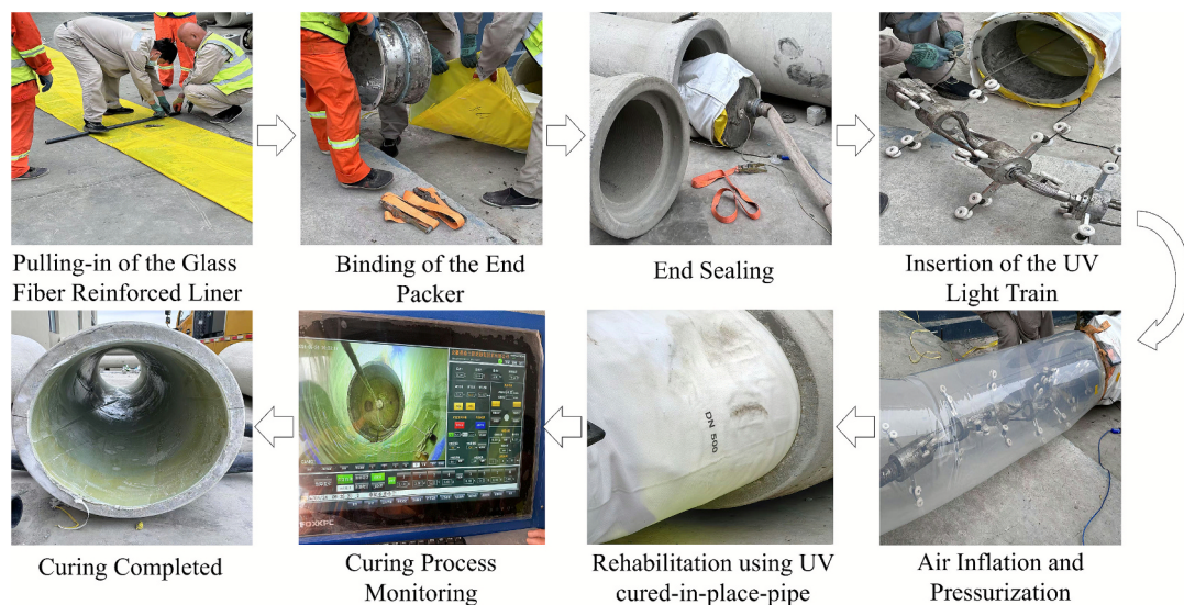
Fig. 2. CIPP Lining Preparation Process.
